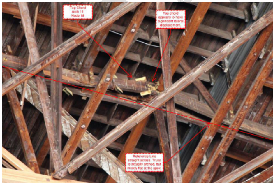
Figure 5. Relative lateral displacement between arch apex and reference line for Hangar 3 single arch.
