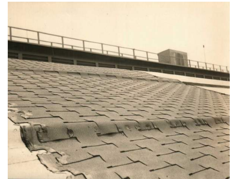
Asphalt shingles documented in 1954 -Seabees Historic Photos
