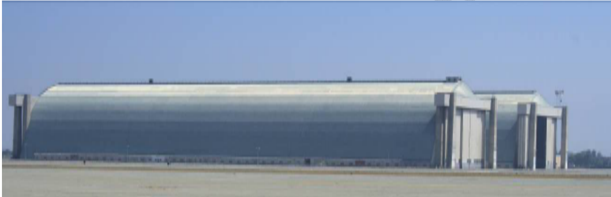
Figure 2. 2013 Hangar 2 (nearest hangar) and Hangar 3.
