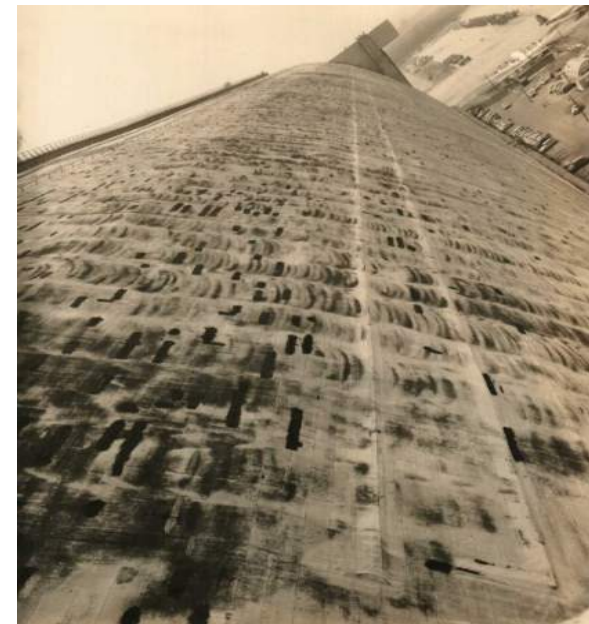
Original roofing system -Seabees Historic Photos
