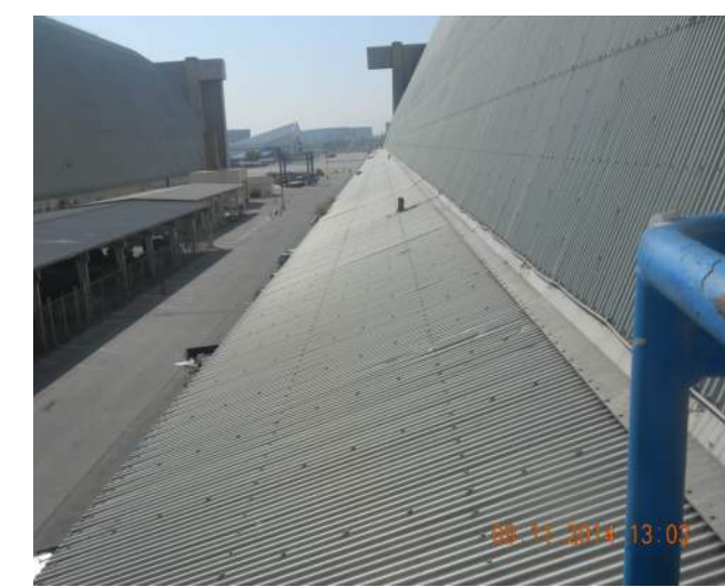
Current aluminum roofing
