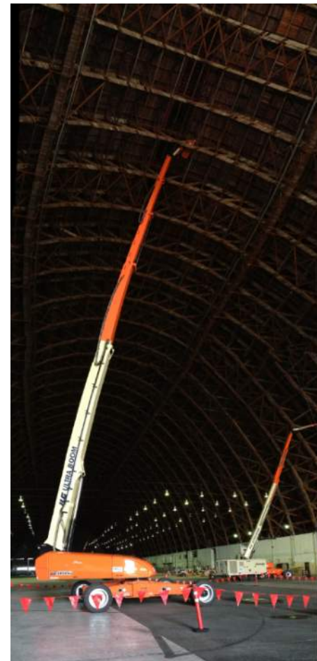
Boom lift used for visual observations
