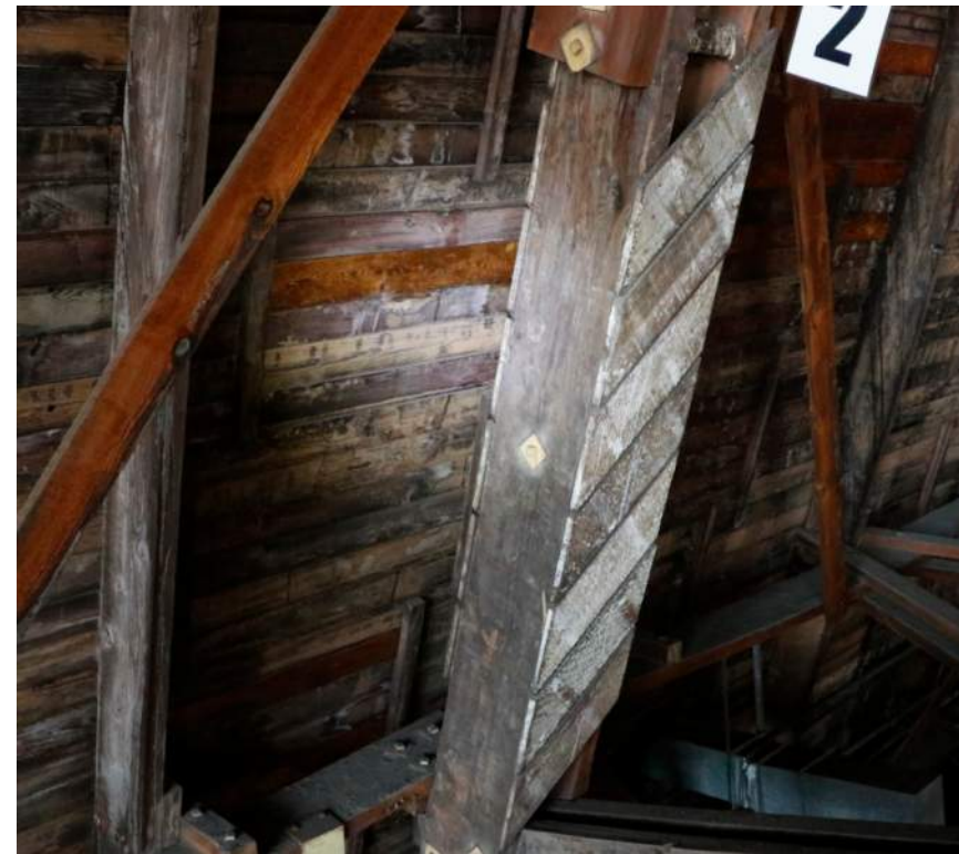
Typical chord member with battens
