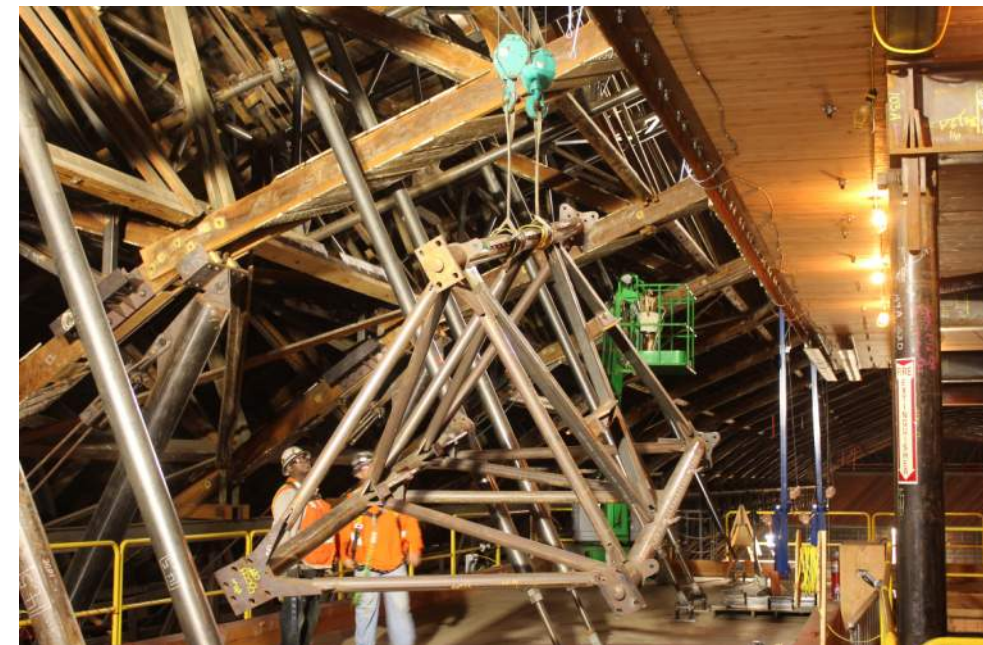
Hoisting exoskeleton segment into place
