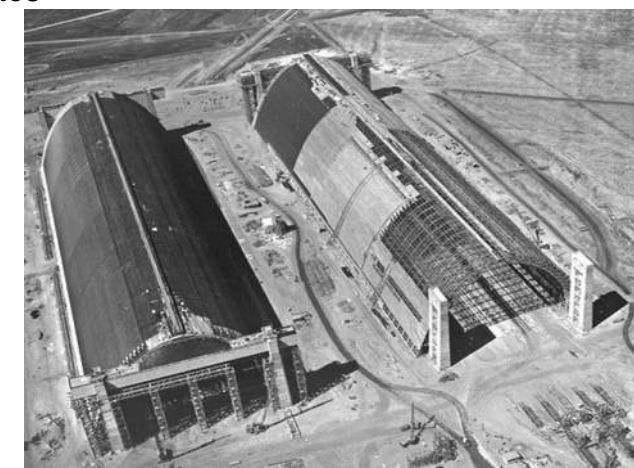
Hangars 2&3 under construction -US Navy Historic Photos
