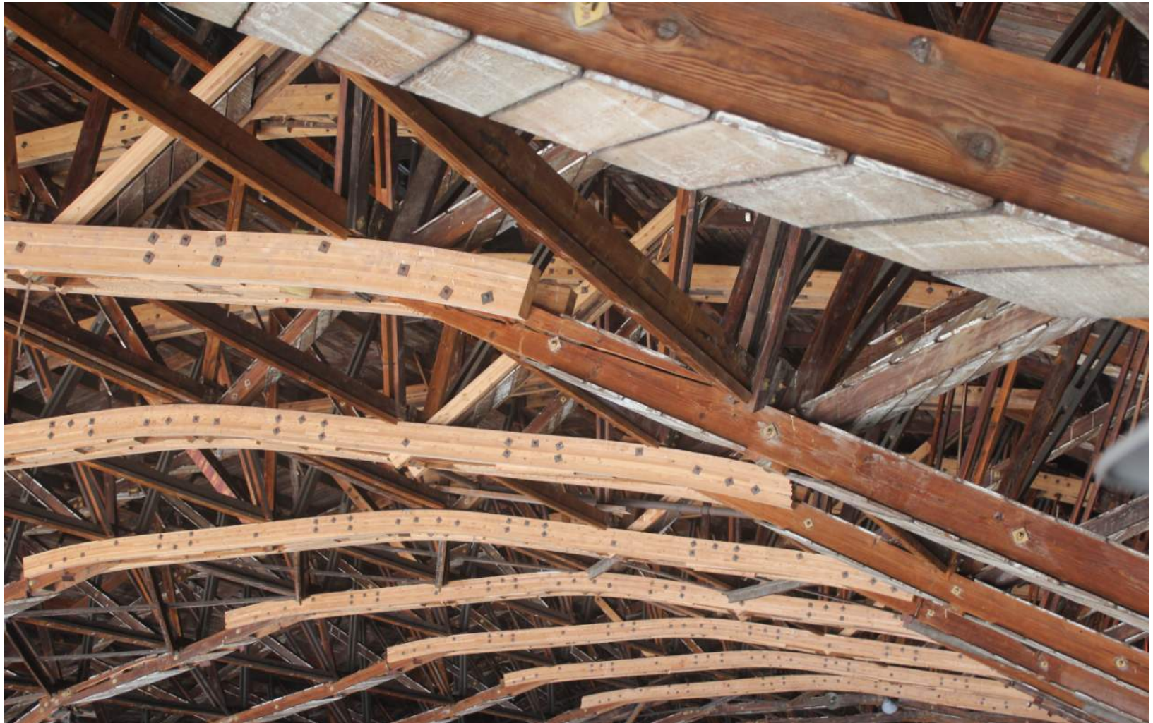
1993 glulam sister repairs to chord members in critical zone
