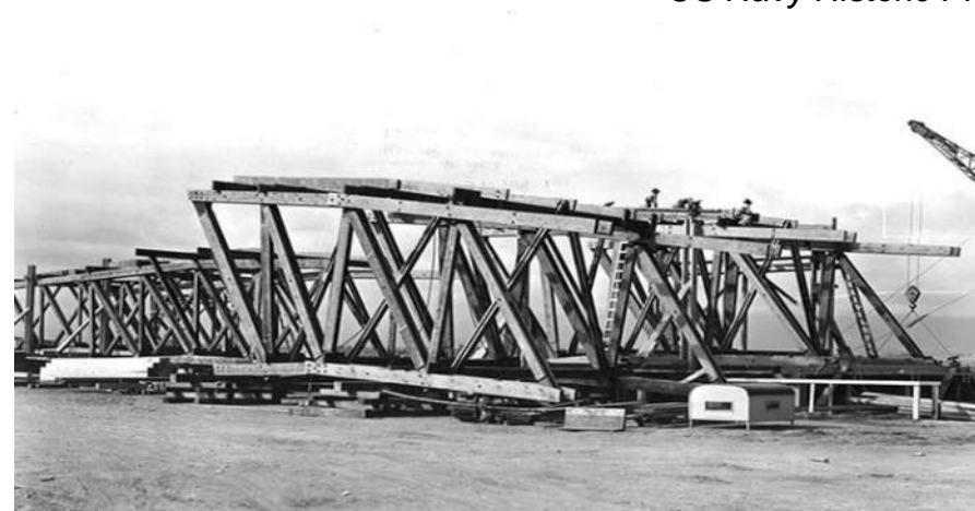
Pre-assembled truss panels awaiting erection -US Navy Historic Photos
