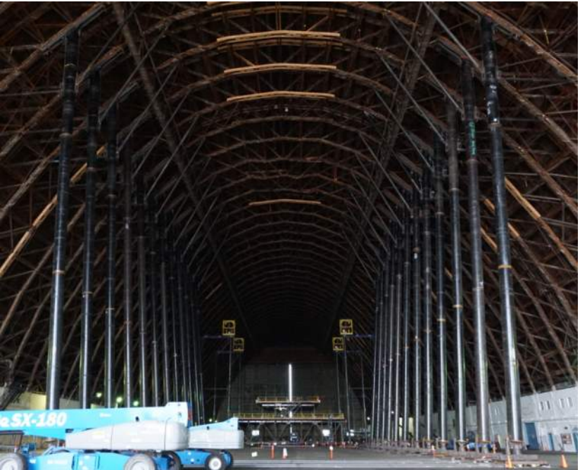
Temporary shores after installation
