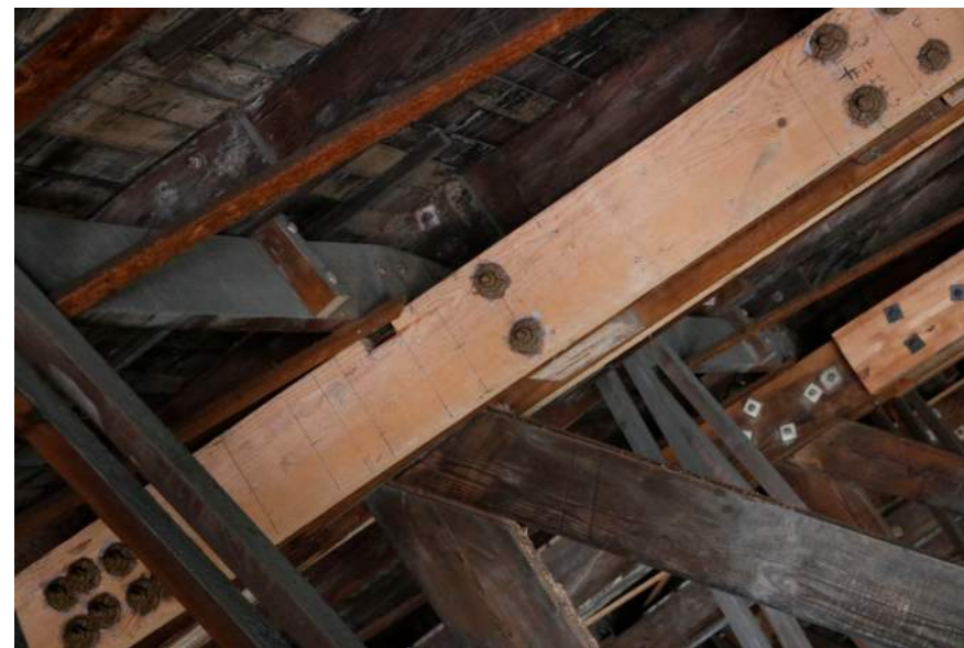
Chord sister repair installed prior to exoskeletons
