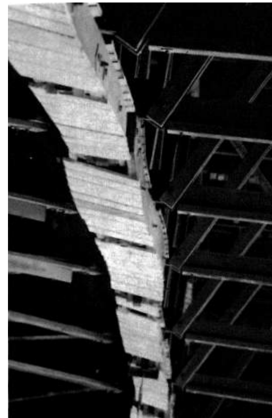
Buckled chords (left) and glulam strongback repairs (right) - "Restoration of Navy LTA (Lighter than air) Hangars", Donal Neal, 1986
