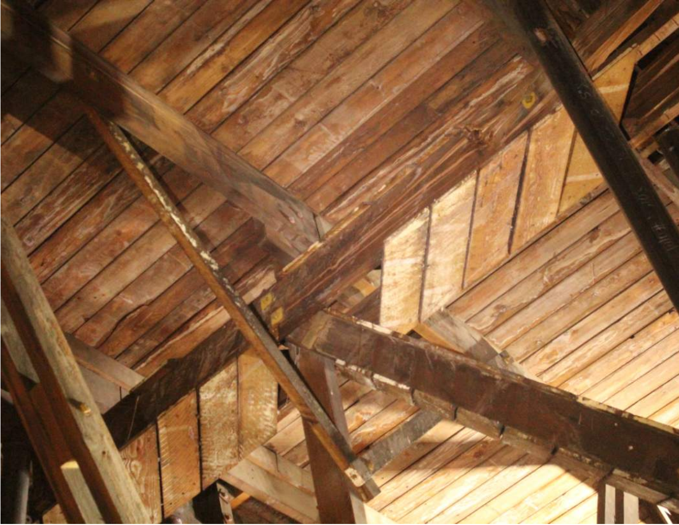
Typical vertical web member with added knee-braces
